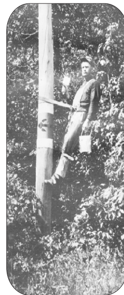
Painting the YT arrow on a utility pole near Cadott
